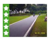
Fully separated facility with one way flows, no side friction, good delineation and forgiving roadsides, 80 km/h
